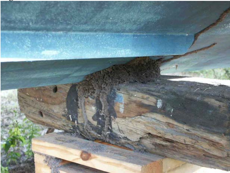
Figure 11. Termite infested boat hull
